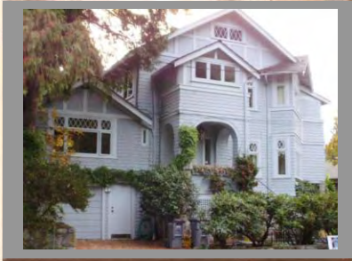
Recent project, replacing wood windows at a heritage house
